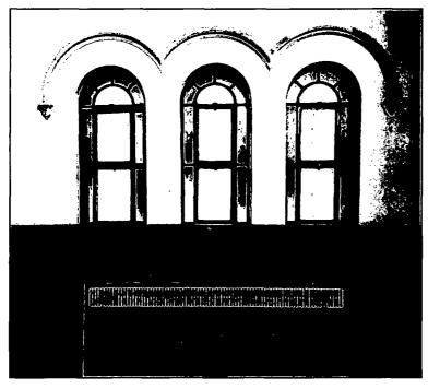
Detail of a window trio along the east aisle. Each window has two operable hopper-type sashes with a plain outer border of amber glass.
