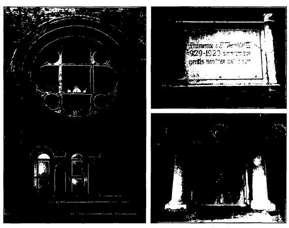
Top left: The east and west facing side windows are round and round arched. All have modern amber and clear stained glass steel sashes. The designs are modern and are set within cast-stone frames.
