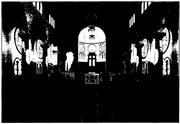
The church's main sanctuary has a tall, barrel-vaulted nave that is flanked by aisles. Colonnades with cast-stone columns and plaster capitals divide the nave and aisles. Facing north.
