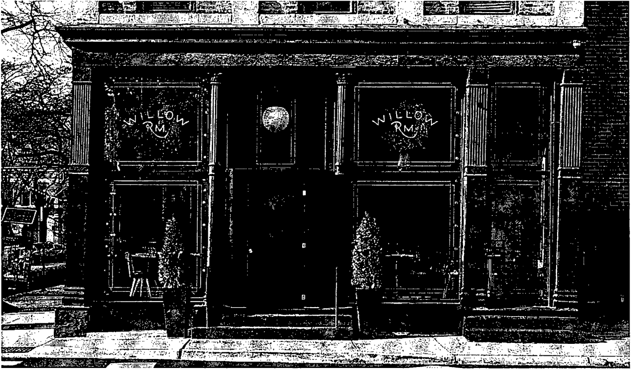
Several of the buildings in the Halsted-Willow Group also have handsome cast-iron storefront columns and lintels. Top: The storefront at 1800 North Halsted Street. Right: A storefront column from 1800 North Halsted.
