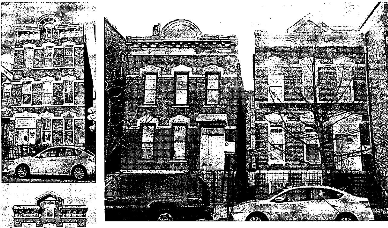
Top: Another version of the two-and-a-half story Italianate style brick cottage incorporates a cornice which forms a parapet above the attic window. Examples include 1840 (left) and 1844 (right), S. Allport St..
